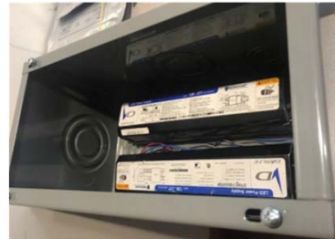
Remote Driver Box (6" x 12" x 4") (only 2 Drivers)
